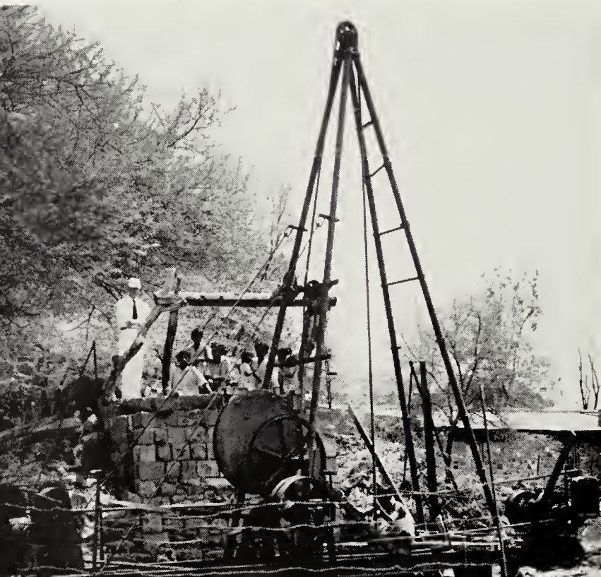
Well-drilling machine, Vadala, India
